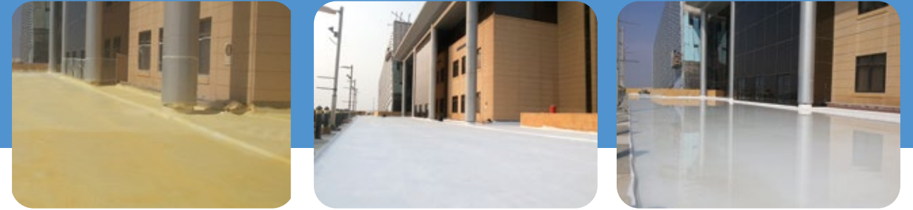
FLOOD WATER TESTING OF THE COMPLETED SYSTEM
