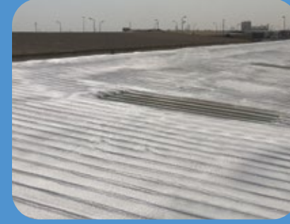
INSULATED STEEL ROOF WITH WATER PROOF SYSTEM
