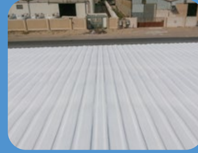
INSULATED STEEL ROOF WITH WATER PROOF SYSTEM
