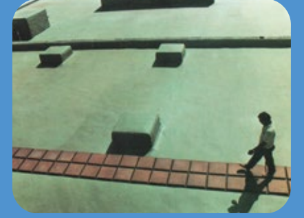
FINISHED ROOF WITH PAVER WALKWAY
