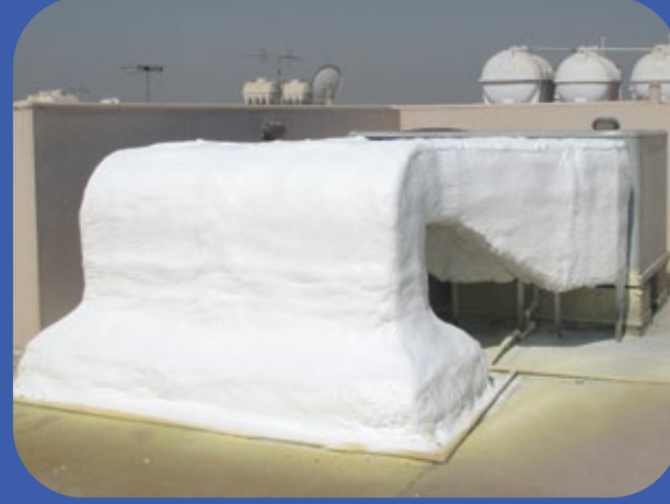
INSULATED AC DUCT
